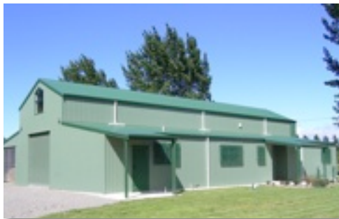
Henley Men's Shed, Masterton
